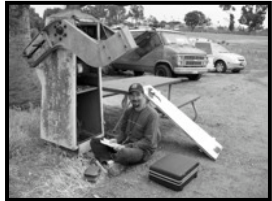
Doug Maywald fixing the crossing signal
