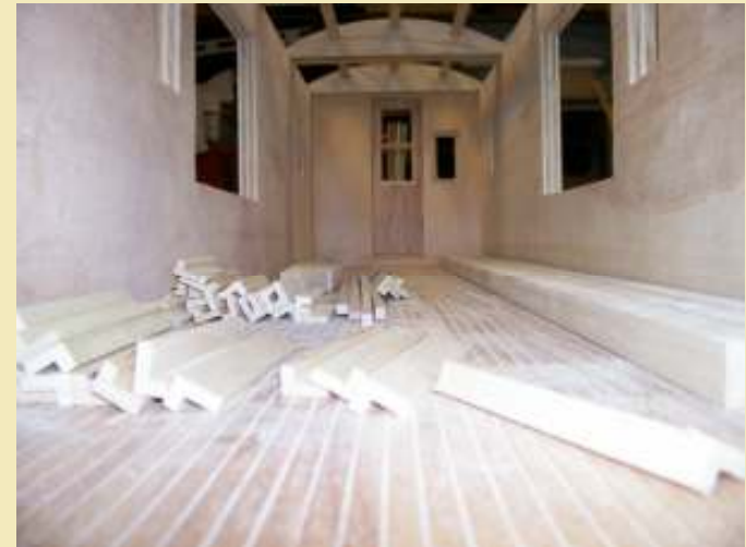
Once closed in, inside & roof construction begins.
