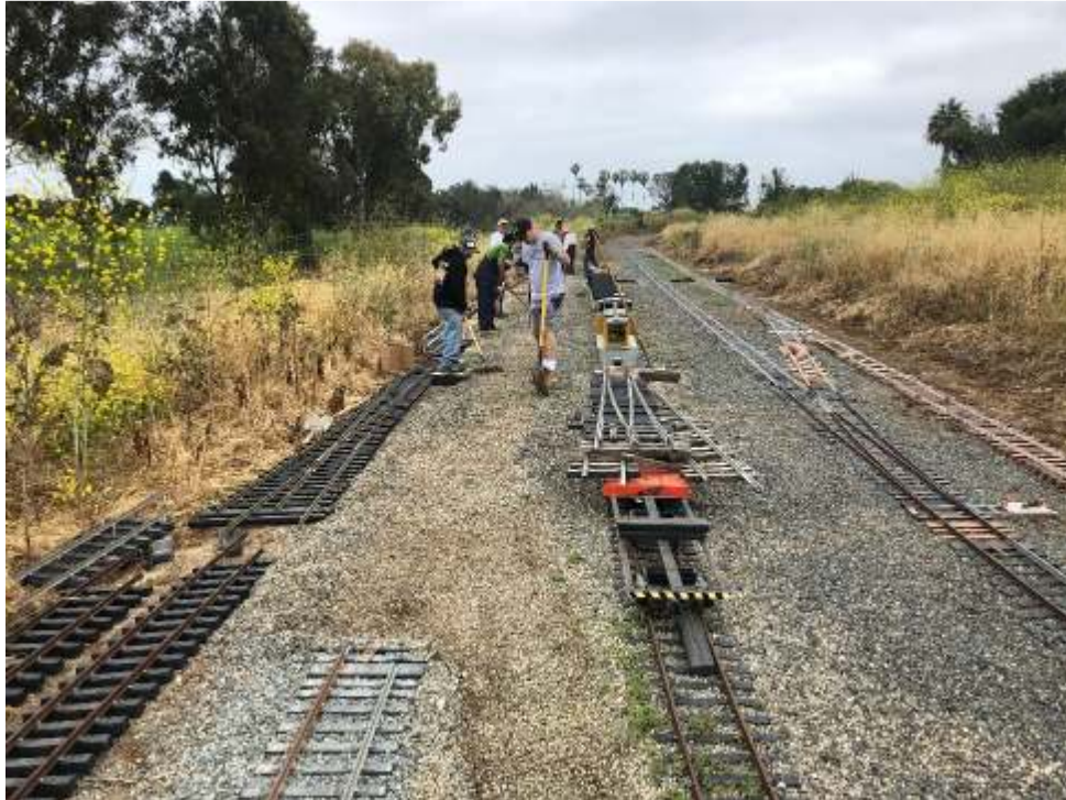
Replacing the Skinner Yard Lead
